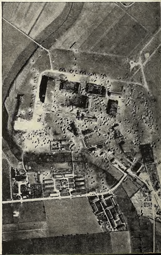
4—Reconnaissance photo after the attack shows the assembly shops, hangars and other structures entirely devastated by the accurate bombing.
